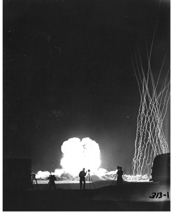
PLK 313-1 - Flare array, generated at t=0 , for photography of airblast Project 9
